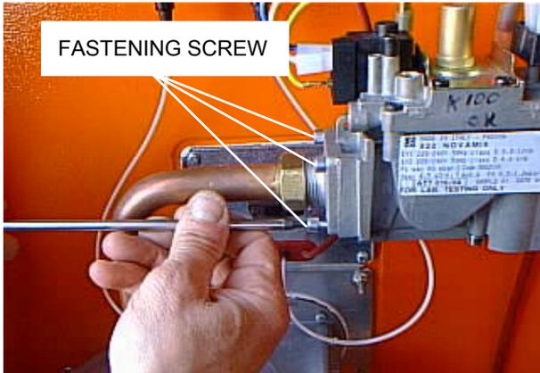
Figure 35 – Gas flange fastening screws
